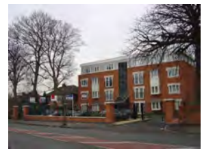
Picture 17 Bad example: Inappropriate in terms of its scale, building line & the loss of the front garden to parking
