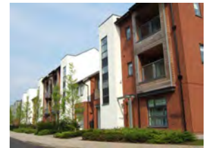
Picture 12 Recess & projection adds interest to this facade
